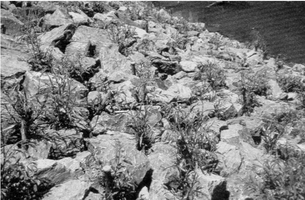
Figure 6. Joint planting system installation
