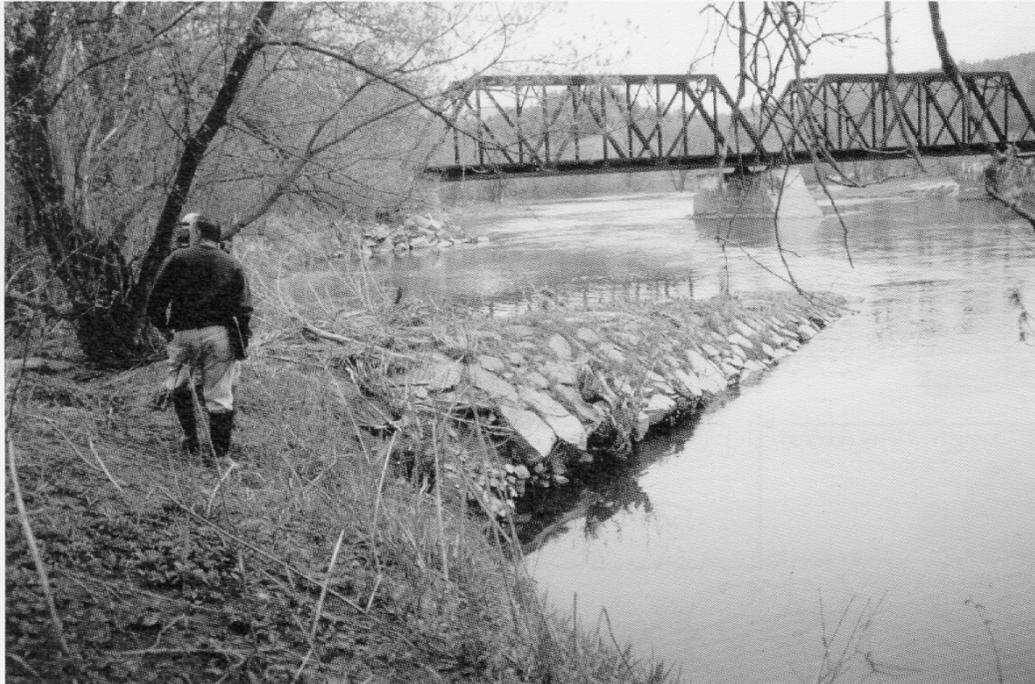
Figure 22. Stream jetty placement for bridge protection
