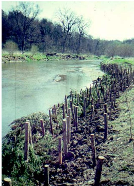
Figure 17. Willow posts on a streambank
