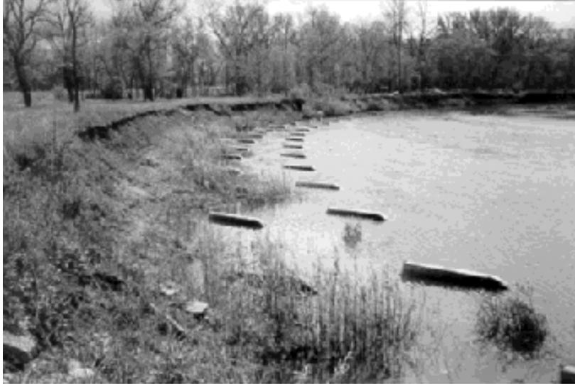
**Figure 26. Replacement of sediment on bank from Vanes**
