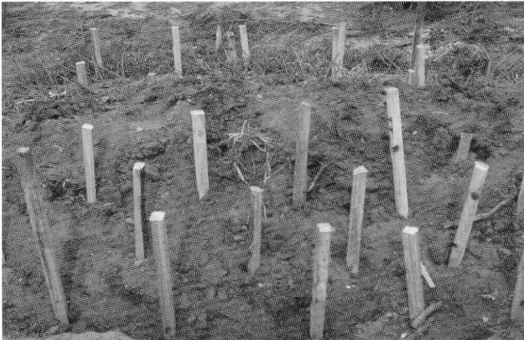
**Figure 5. Live stake installation**
