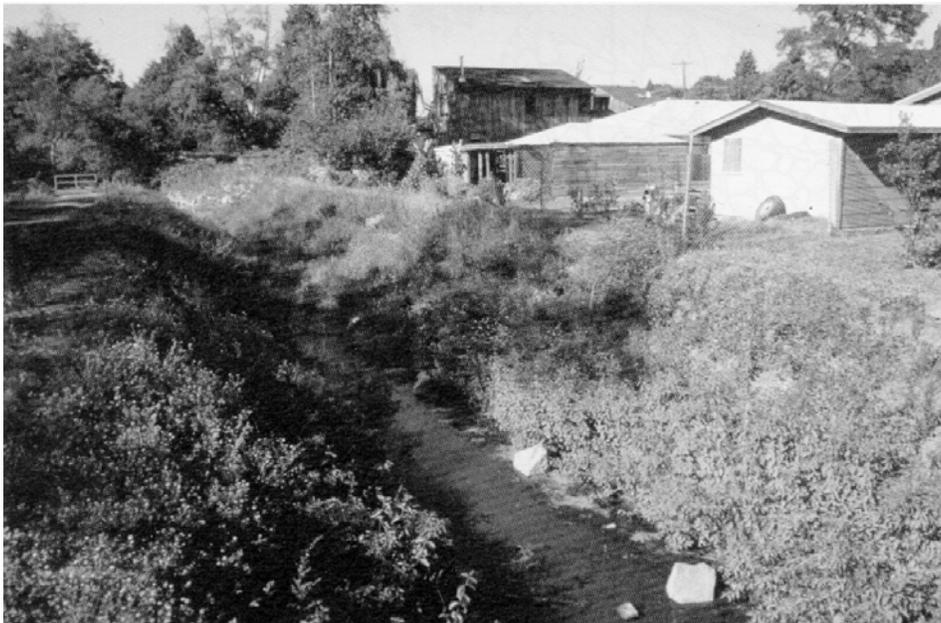
**Figure 29. Vegetated geogrid two years after installation**
